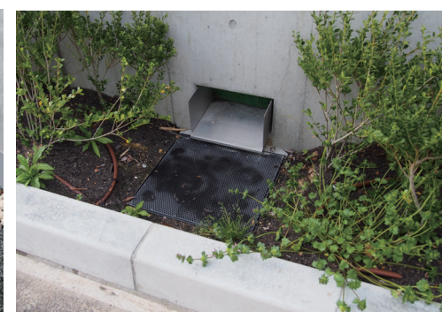
An open spout discharging runoff to the sidewalk
