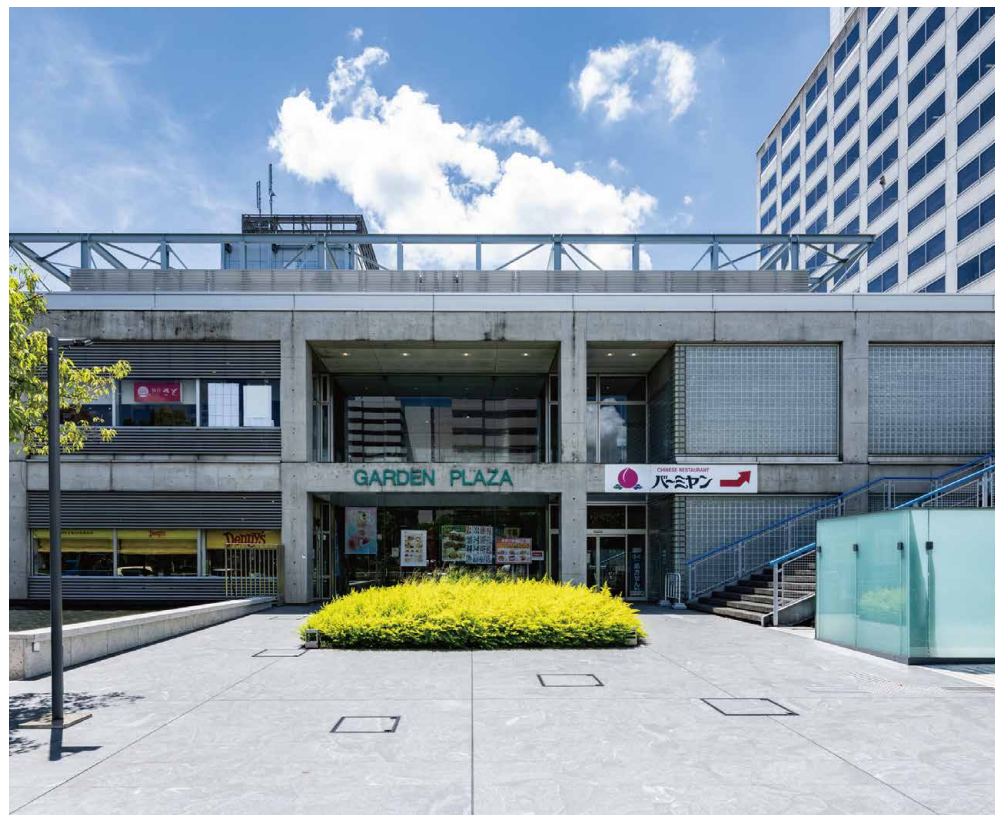
After: Visibility considerably improved by clear demarcation of bicycle parking and thinning out of trees
