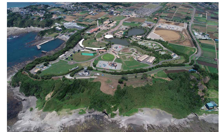
Construction in progress as of July 2022
