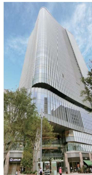
Exterior of Hibiya Mitsui Tower, Tokyo Midtown Hibiya
