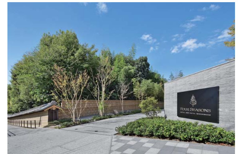
Main Entrance Gate In order to harmonize with the roofed-mud wall of the adjacent Temple, natural ashlar stacking was used for the Entrance Gate. And the Security Room is contained within the walls.
